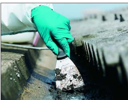
Wet the debris again if you find dry material, avoid creating a slurry
